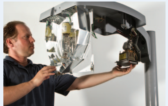
Remove the existing HID reflector system and ballast tray.
