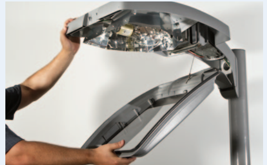
Unlatch and remove the existing door.
