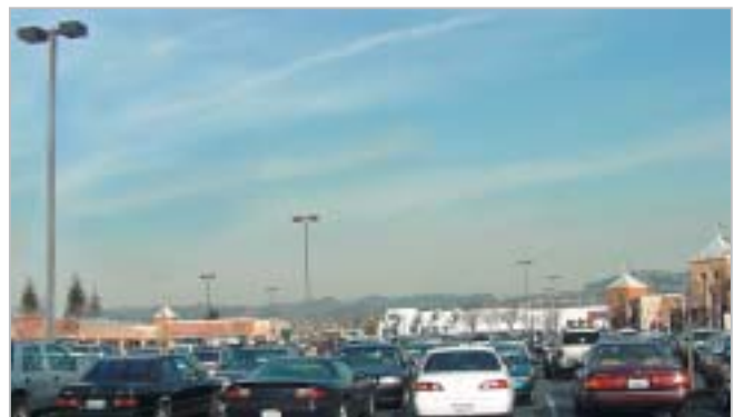
Permitting the application of taller poles will allow for wider spacings resulting in significantly reduced energy consumption.
