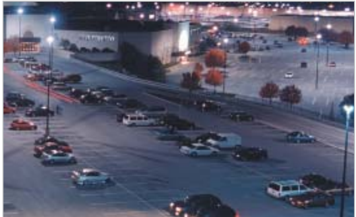
Older sites often have light levels which are substantially below contemporary standards.
